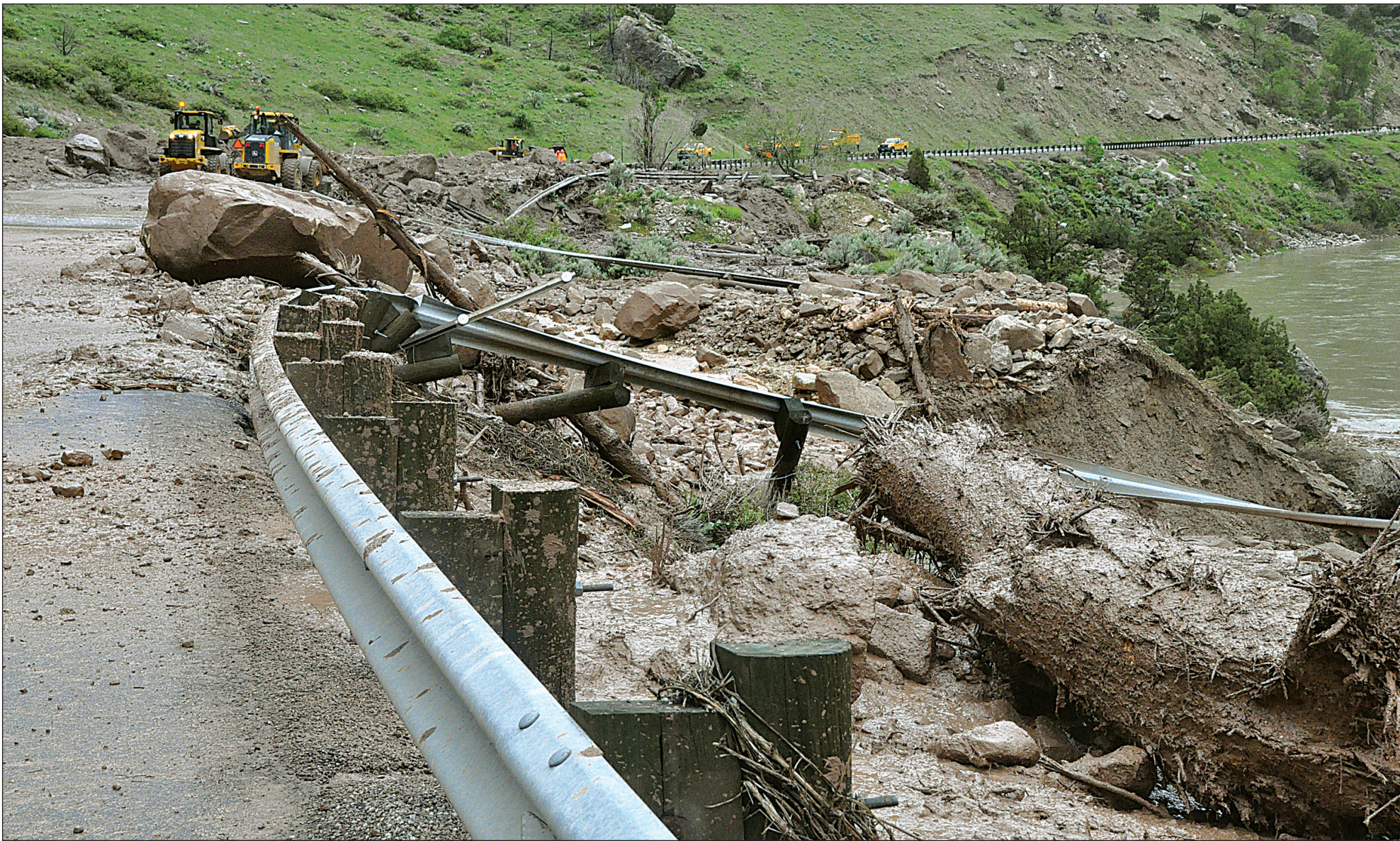
More than 300 yards of guardrail were destroyed in Sunday's rock slide in Wind River Canyon. Here, crews from WYDOT work to move tons of mud, rocks, trees and other debris that roared down the canyon wall toward the river. – Cindy Glasson photo
