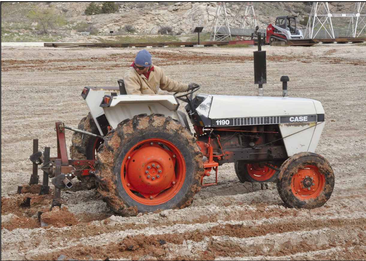
A Tommaron, Inc. employee plows one of the cooling ponds in Hot Springs State Park to help dry the soil and prepare for the application of sand and a polyethylene pond liner. Four cooling ponds were drained and will be refilled as part of the project.
