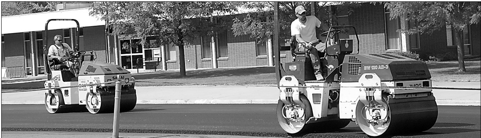
Two equipment drivers for a subcontractor working on the Arapahoe Street Waterline Replacement project roll the newly installed asphalt near the Hot Springs County Library. – J.D. Stetson photo
