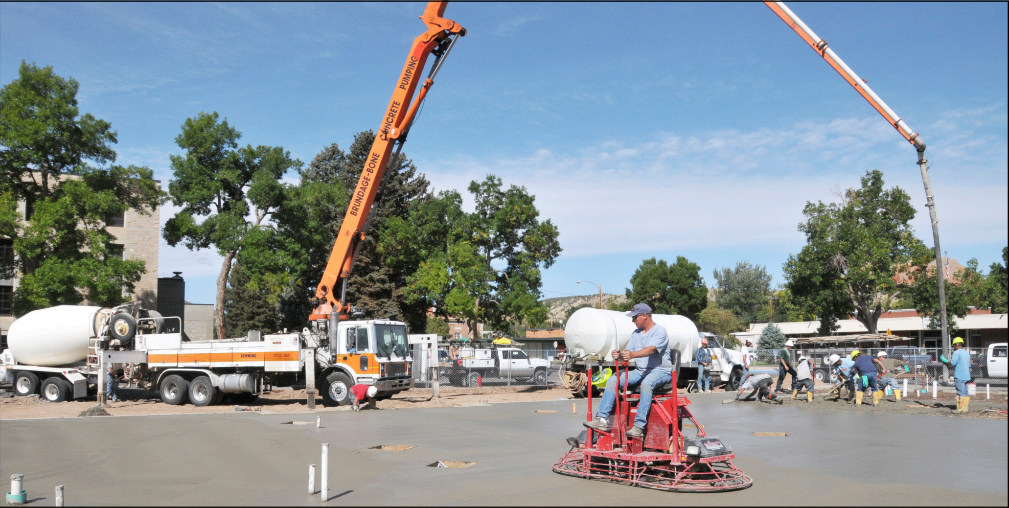
Brian Piper with Construction Concepts rides a power trowel, the modern way of smoothing concrete at the site of the new Government Annex building on Tuesday. At right, other workers spread and leveled the cement after
